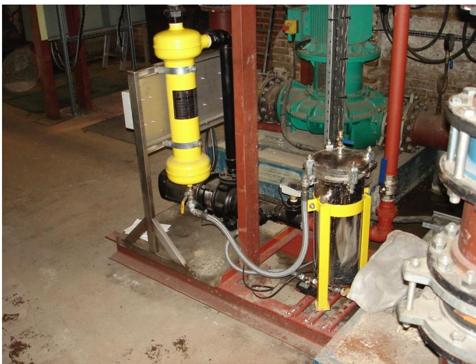
New sidestream filtration unit. This is a cyclone type cleaner; dirt collects in a bag within the container on the right and requires periodic emptying. The green pump seen at the rear is one of the two main cooling tower pumps.
